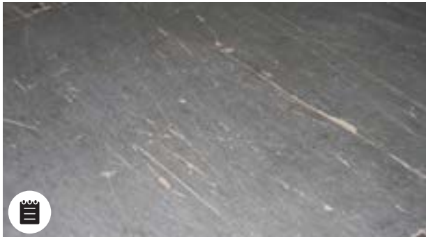
Flooring: Slight deformation, superficial wear
