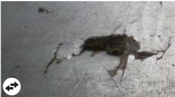
Flooring: Deformations or perforations within economic repair
