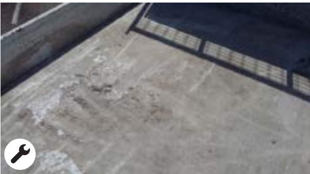
Trace of concrete or chemical product covering \geq 1/4 of the surface of the bed
