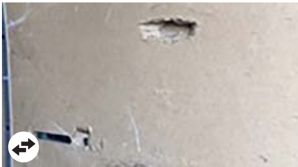
Wood internal protections: Impacts > 2 cm, torn panel, panel missing (excluding door upper panels)
