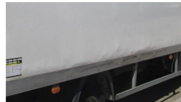
Fibreglas side panels: Deformation on lower part, length of > 1\text{ m} NB: Replacement of the front panel of the underbody requires removal of the underbody.
